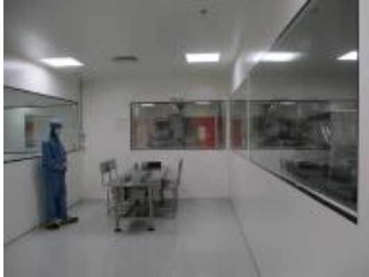
Strip area- packing area- ground floor.JPG
